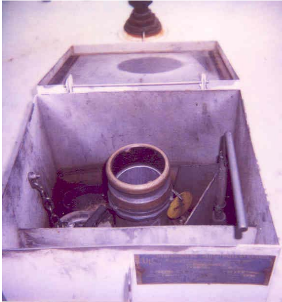
Unloading Piping : 3 or 4 inches
